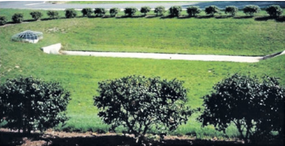
Proposed temporary dry basin used all over the world with gentle slope retaining no water.
